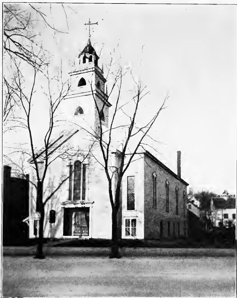
THE CONGREGATIONAL CHURCH AT TILTON, NEW HAMPSHIRE
